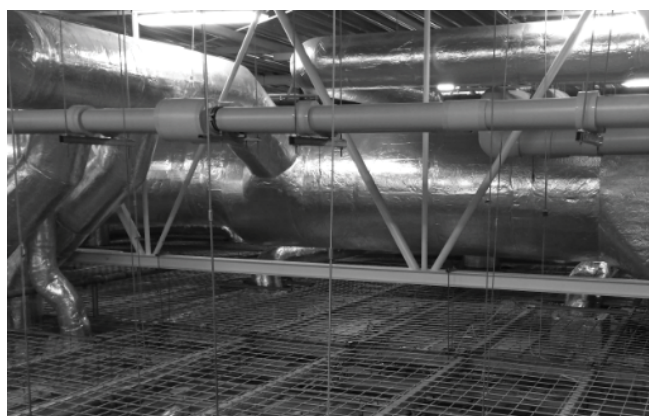
Photo 1. a) High frequency welder, b) air condition main supply duct (the secondary source of electromagnetic field) placed above the suspended ceiling
